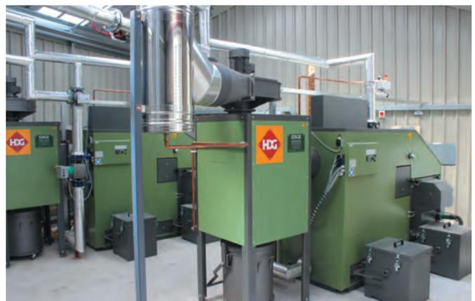
The Shrewsbury Club has constructed an energy centre, which houses two 199kW biomass boilers that produce all of the site's heating and hot water
