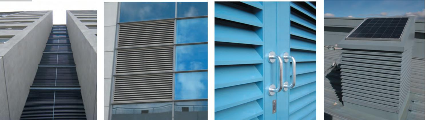
GDL's products are divided into four segments, grilles, diffusers, louvres and natural ventilation (intelivent). Examples of GDL's work are pictured here
